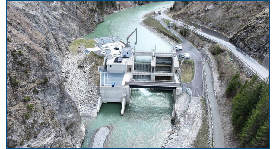
The recently constructed dam of the new Gemeinschaftskraftwerk Inn (GKI) power plant, situated on the Upper Inn River in the border region between Austria and Switzerland. The GKI must comply with strict environmental regulations.
