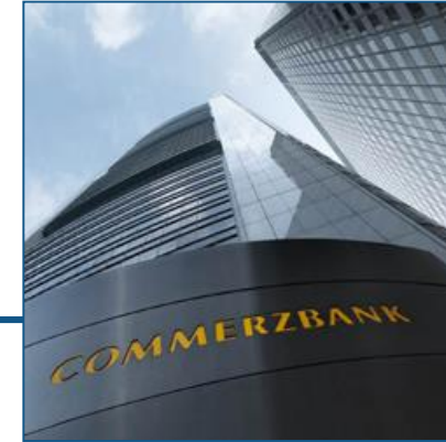
Commerzbank headquarters in Frankfurt.
